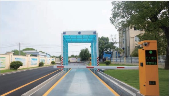
Unattended floor scales for hazardous waste intake and outbound shipments
